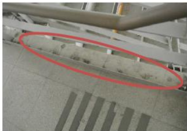
樓梯拖淨、灰塵掃掉清掉
